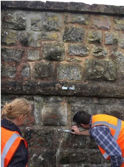
Figure 7. Vertical crack on the abutment wing wall.
