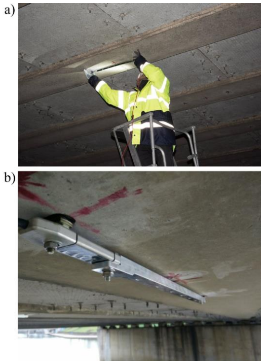
Figure 2. Sensor installation: (a) ESR installing sensors on the soffit of the main girder, (b) close view of the installed sensor.
