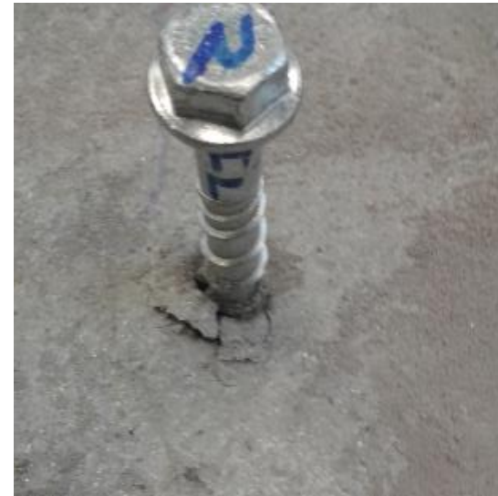
Complete pullout failure
