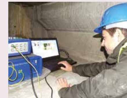
António Barrias (ESR11) testing distributed optical fiber sensing system
